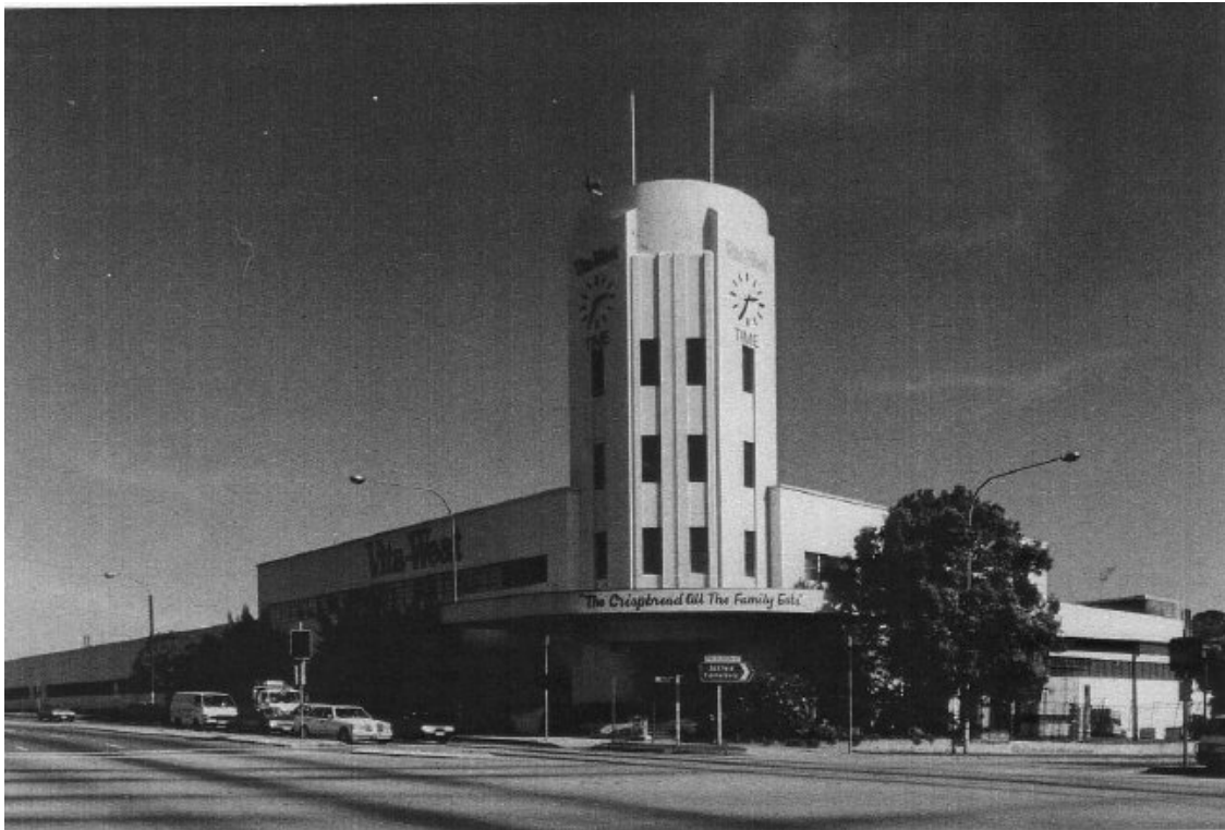
Figure 4.80 Former Vita Weat/Peak Frean Factory in the 1980s. (Source: NSW State Heritage Inventory)
