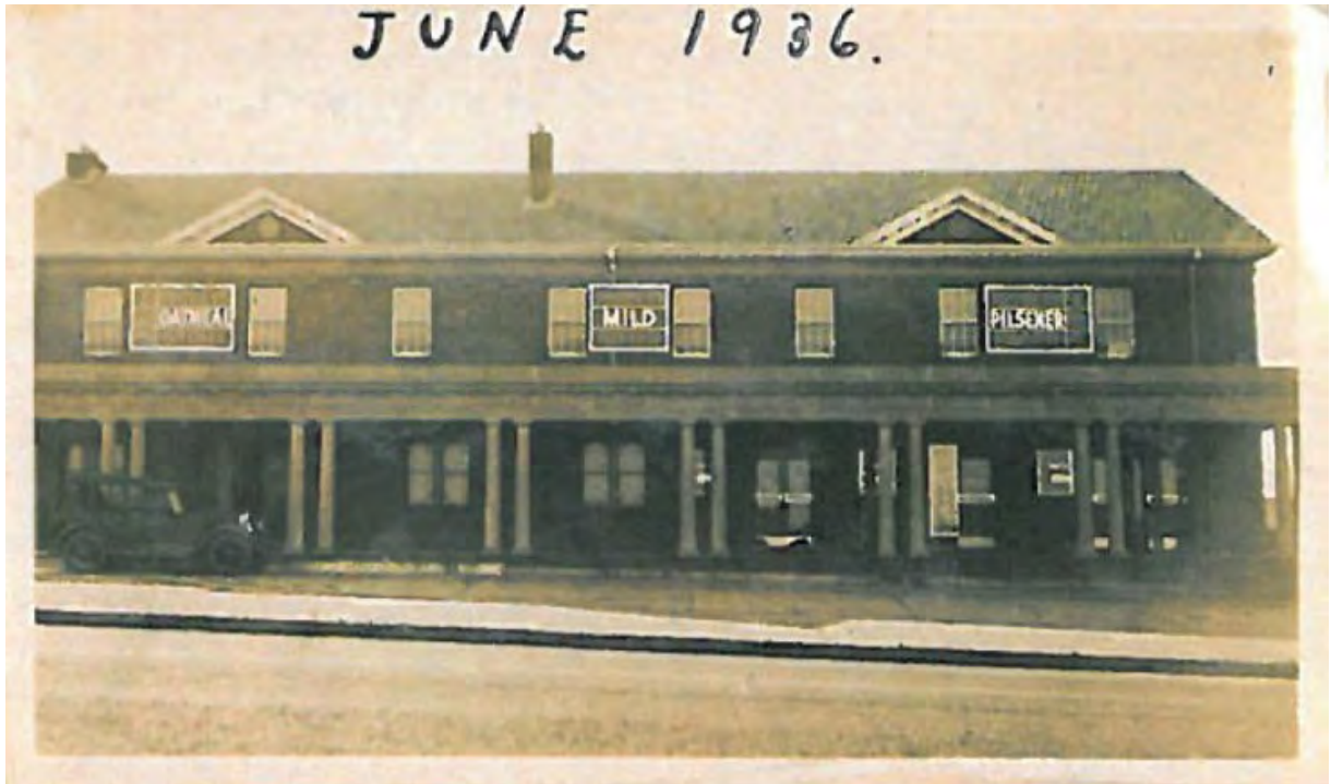
Figure 4.9 The newly re-constructed Wentworth Hotel, June 1936. (Source: Noel Butlin Archives)
